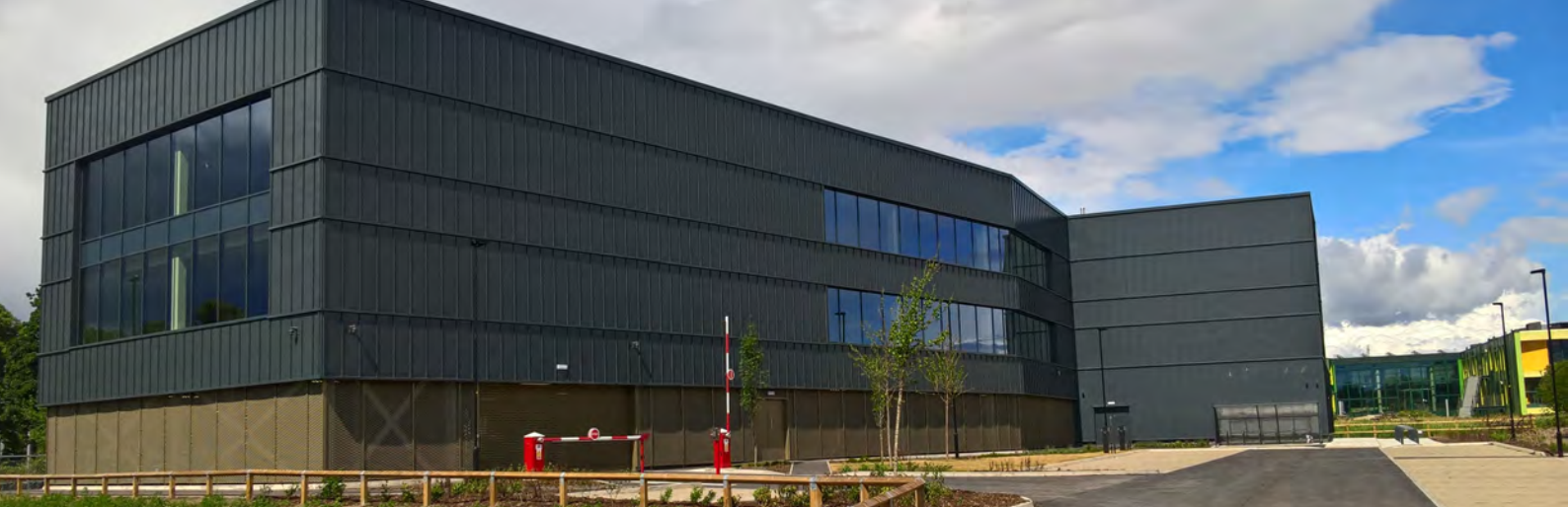
Elizabeth Garrett Anderson Building, Nottingham Science Park
