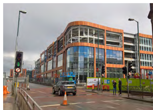
New library and car park, Nottingham
