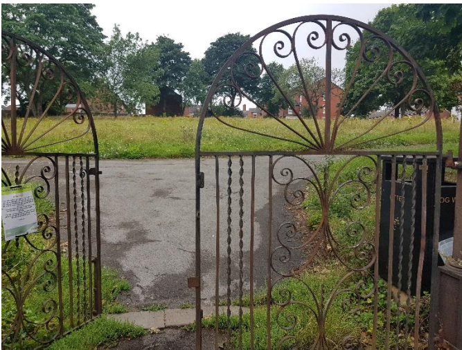
Poor quality entrance at Basford Road Burial Ground
