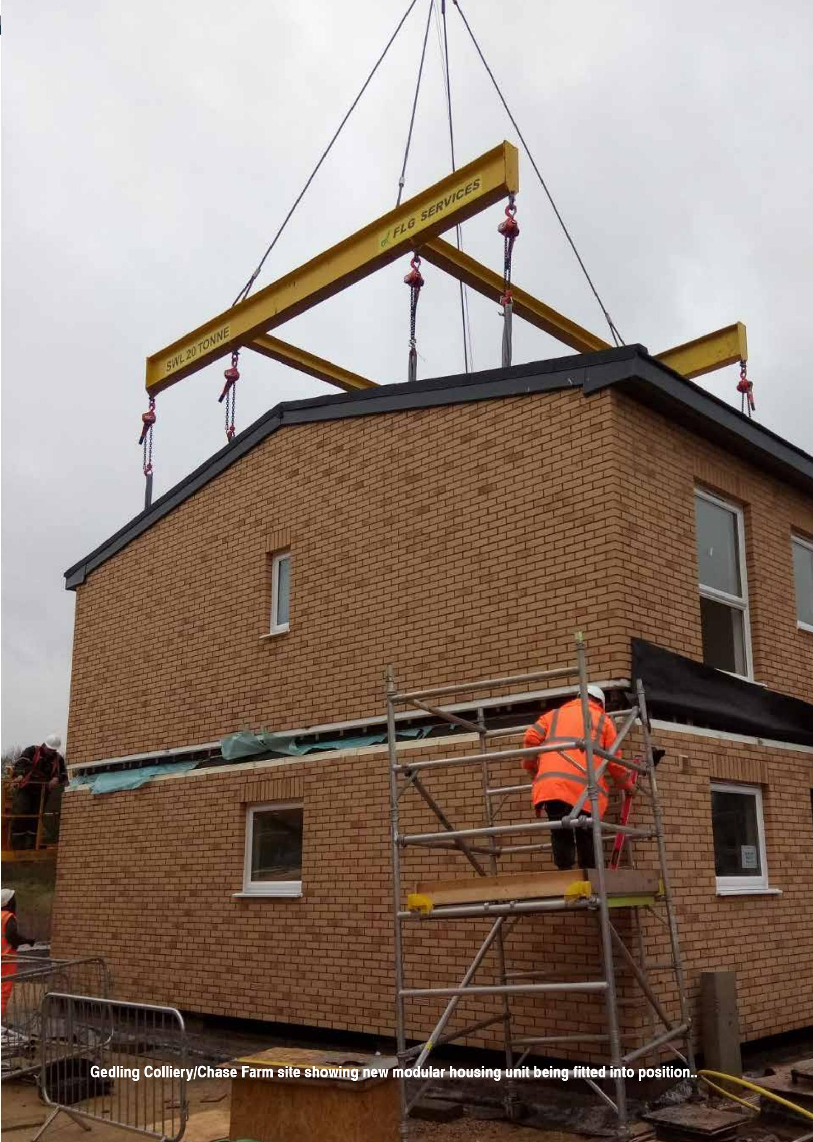
Gedling Colliery/Chase Farm site showing new modular housing unit being fitted into position..
