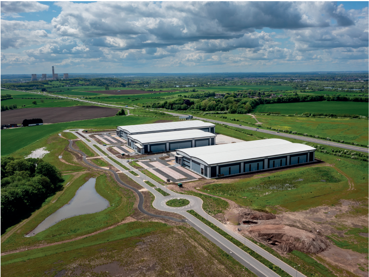
View of Fairham Business Park looking west towards Ratcliffe on Soar Power Station.
